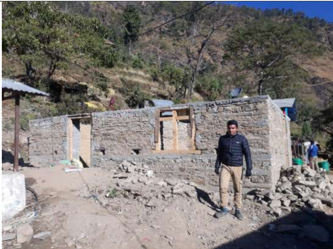
Suraj's under construction home.
